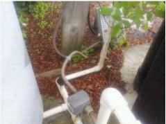
The sub panel is damaged and is missing the cover plate. A safety hazard is present. Have a licensed and insured electrical contractor properly repair or replace the sub panel and install the missing cover plate.
