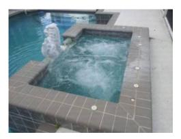
Minor cracks are noted at tile surround. Properly re-grout cracks at tile.
