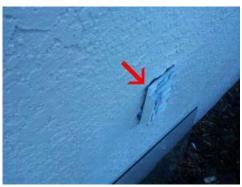
Stucco wall at rear of house at second story has expansion cracks. These types of cracks will allow water to penetrate into wall. Properly seal all exterior cracks to prevent water penetration, paint to match.
