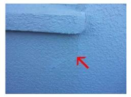
Small opening(s) noted at wall penetration where outlet is present at left side of house. This type of opening will allow water and insects to enter the home. Properly seal any / all openings at wall penetrations.
