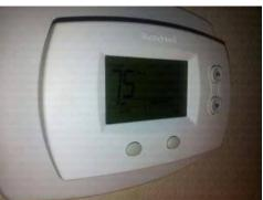
RETURN AIR TEMPERATURE: SUPPLY AIR TEMPERATURE: AIR TEMPERATURE DROP: SYSTEM CONDITION: DUCTWORK TYPE: Approximately 74 degrees. Approximately 60 degrees. Approximately 14 degrees.
